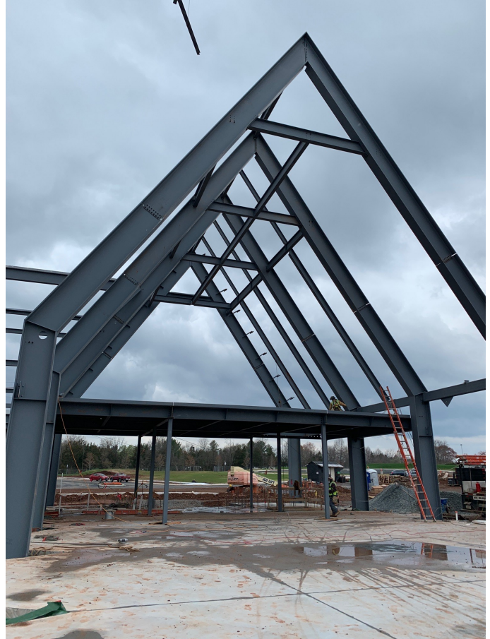
STEEL ERECTION AT NARTHEX
