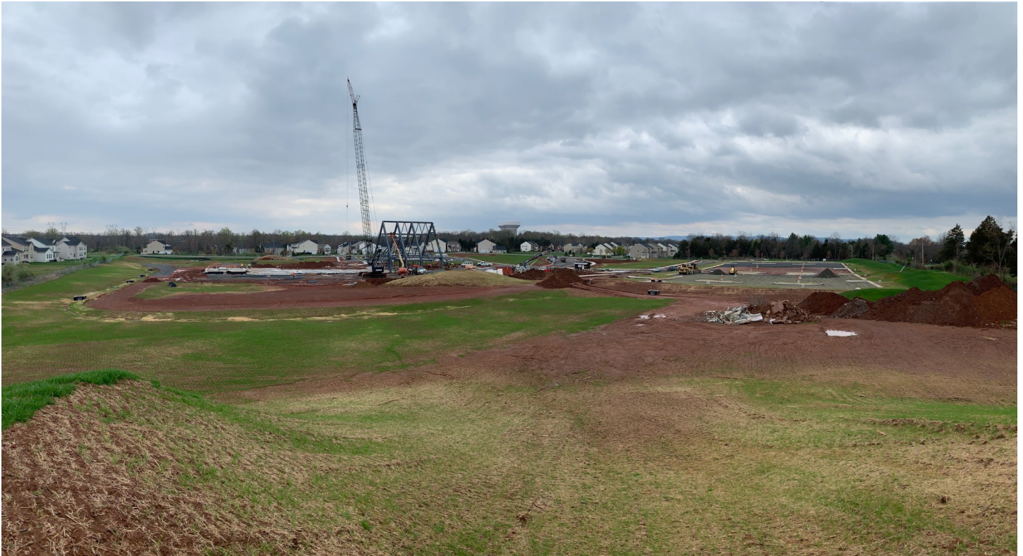
PANORAMIC VIEW OF SITE FROM NORTH EAST CORNER
