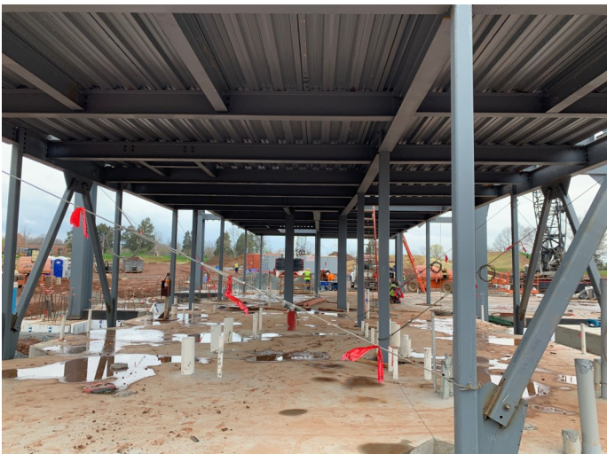
STEEL ERECTION AND DECKING AT SOUTH SERVICE WING
